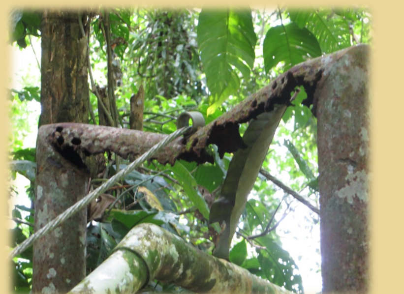
Figure 1. Degraded Metal Support
